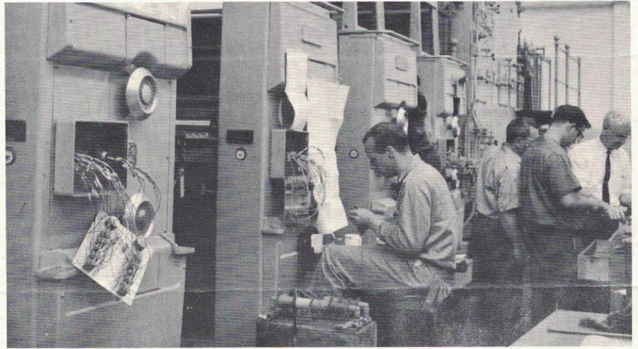
Mr. Shelton adjusts electrical circuits to prepare units for use.
