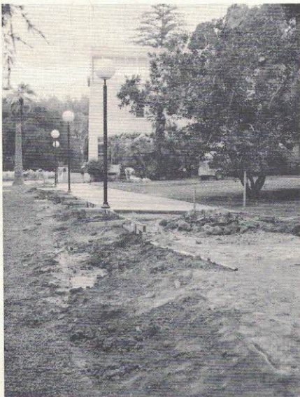
Even in the construction stages the ultra-modern walk is very beautiful.
